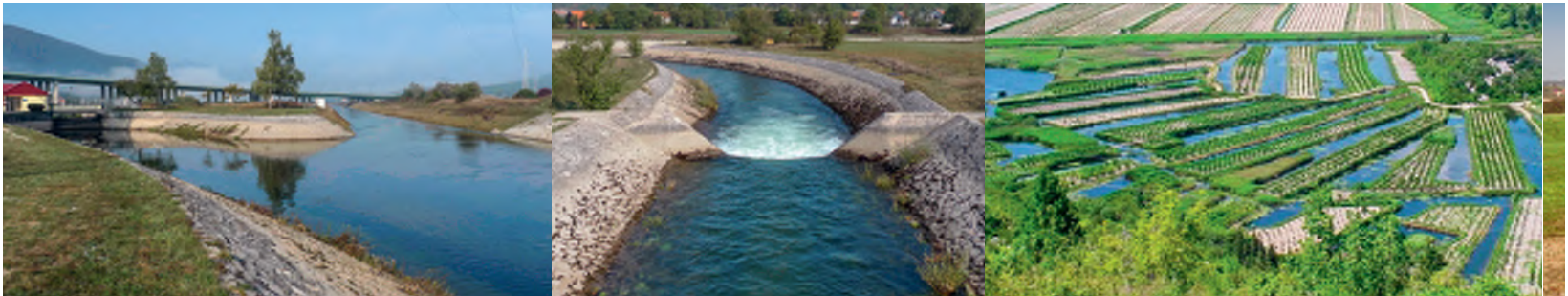
Senj Hydropower System
